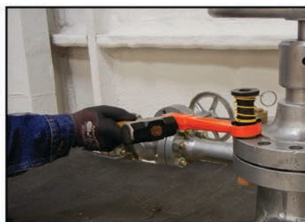
Screw the HAMMERTIGHT wrench retainer onto the stud. At least two threads of the stud must be engaged into the retainer.
