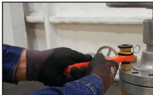
Leaving the HAMMERTIGHT wrench retainer engaged on the stud, lift up on the wrench to reposition.
